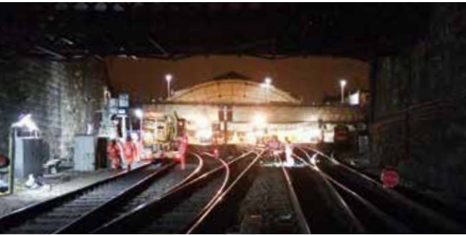
Queen Street Tunnel
